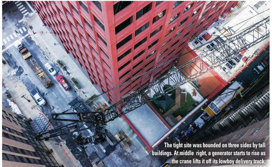
The two outriggers at right sit on the vaulted sidewalk. The engineered mats plus shoring in the building's basement provided solid support. The mat in the left foreground includes a steel plate to protect underground utilities.
